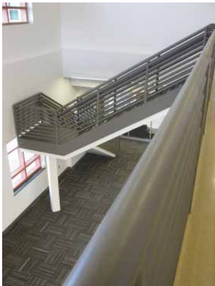
Stairway to upstairs classrooms
