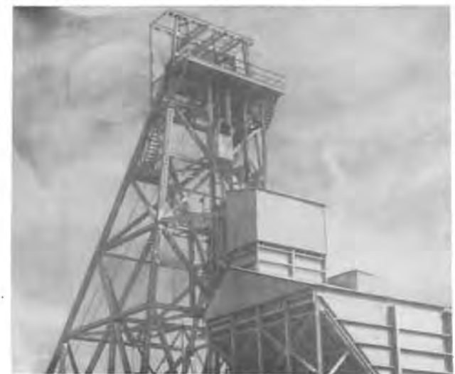
THE "GALLOWES" . . . in mining vocabulary refers to a mine shaft headframe, such as this one, pictured below, located at the modern U. S. Potash Mine near Carlsbad.
